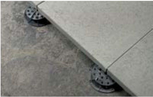
Terrace Slab uses pedestals for rooftop applications.
