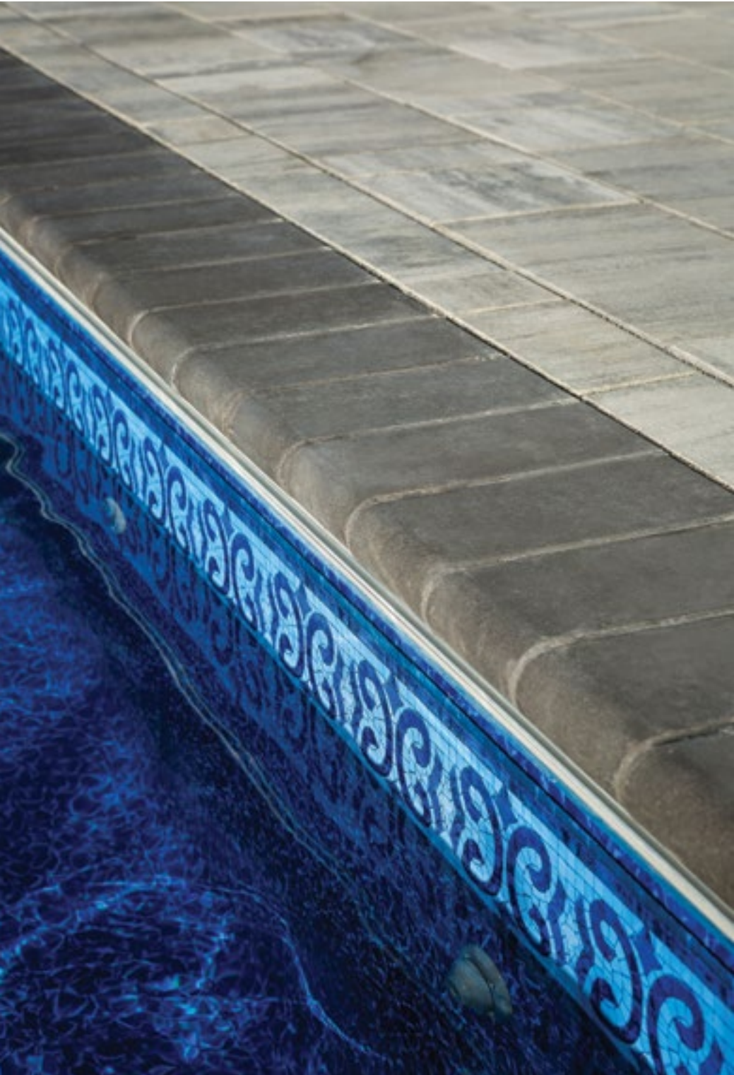
Bullnoses pavers are primarily used as a border paver around pool decks or as a step cap.
