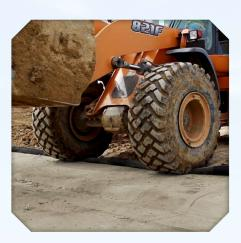
DuraWattle is made to be driven over by heavy equipment without any change to its overall effectiveness. Unlike traditional wattles, the inner core of DuraWattle is non-permeable and does not take on water. The plastic sealed foam core gives the barrier its height and helps maintain its shape after being driven over by heavy traffic.
