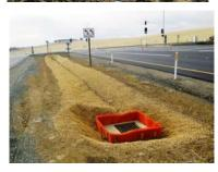
Minimization of off-site sediment loss is achieved with a combination of BMPs. Here and erosion control blanket is used in combination with Drop Guard.
