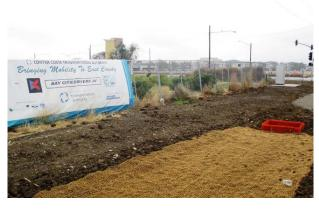
management practice system for site sediment control. Highly sustainable zero waste solution, the system is made from recycled, reusable and recyclable HDPE.
