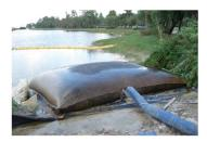
This letter certifies that our Dewatering Bags, manufactured by L&M Supply Co., are made with 8 oz. non-woven geotextile fabric. Our Filter Bags/Dewatering Bags are inert to biological degradation and resists naturally encountered chemicals, alkalis, and acids. The stitching is a durable, double thread chain stitch. Custom Sizes are available.
