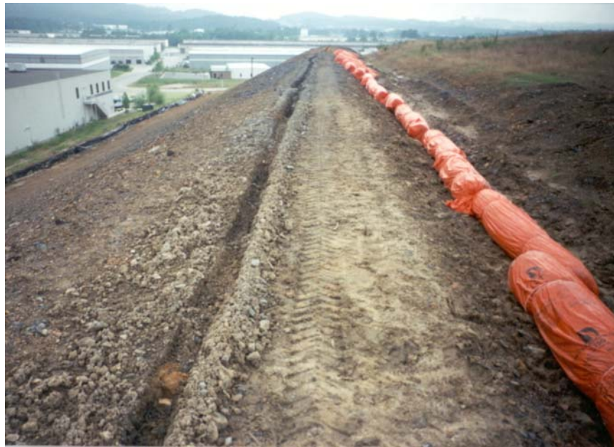
Slope Step Three – Prepare the Anchor Trench
