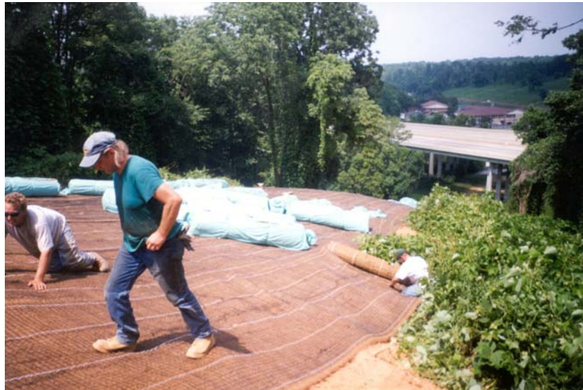
Slope Step Five –RECP Deployment
