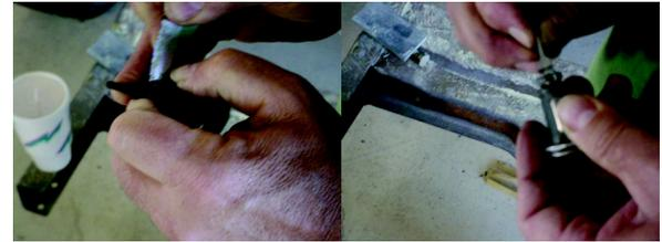
Remove pin from stock lock cylinder. This is done by depressing the spring with a pocket knife or small screwdriver, then slide pin out.
