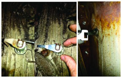
When feeding the lock cylinder back into the door, do so at an angle and make sure the lock arm goes into the rectangle shaped opening in your Altman Easy Latch locking mechanism. Secure it to the door using the U-shaped clip you removed earlier.
