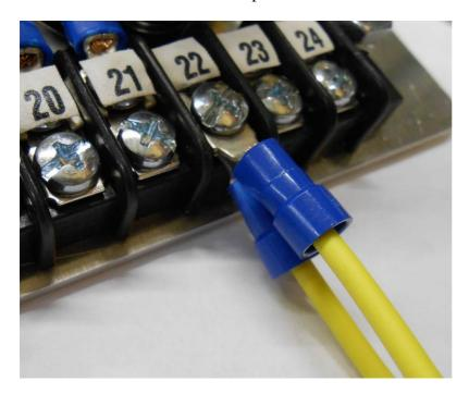
In the picture above, you will notice that the first wire installed on Terminal #22 is the Rear Left Turn wire and it is installed "Face Down." The second wire installed on Terminal #22 is a part of the Turn Signal Switch Pigtail and it is installed "Face Up."
