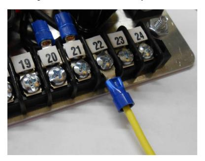
As you continue adding wires to the Power Panel, you will eventually find that a second wire may need to connect under the same numbered screw. If you installed the first terminal "Face Down" it will be simple to install the next terminal "Face Up." It should not be necessary to install more than two terminals under the same numbered screw on the panel.
