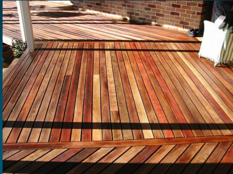
Timber Seal used on a deck
